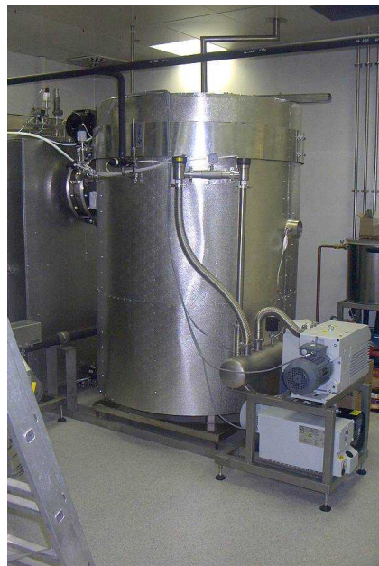
condenser and vacuum pump station
