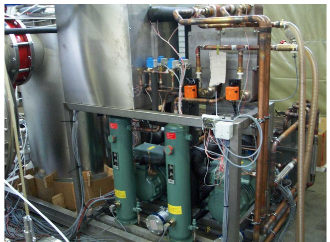
2-stage Bitzer cooling machine
